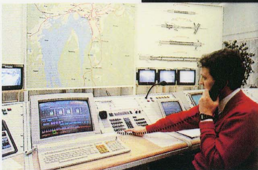
This traffic control centre for Oslo employs advanced systems for managing vehicle movement in the Oslo Tunnel and large parts of the main highway system around the capital.
